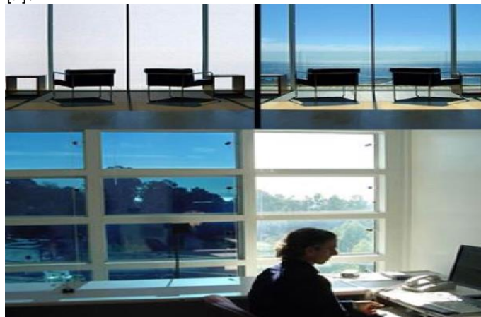
Figure 1 Two examples of electrochromic smart windows each are having both the fully colored and the bleached state [3].
